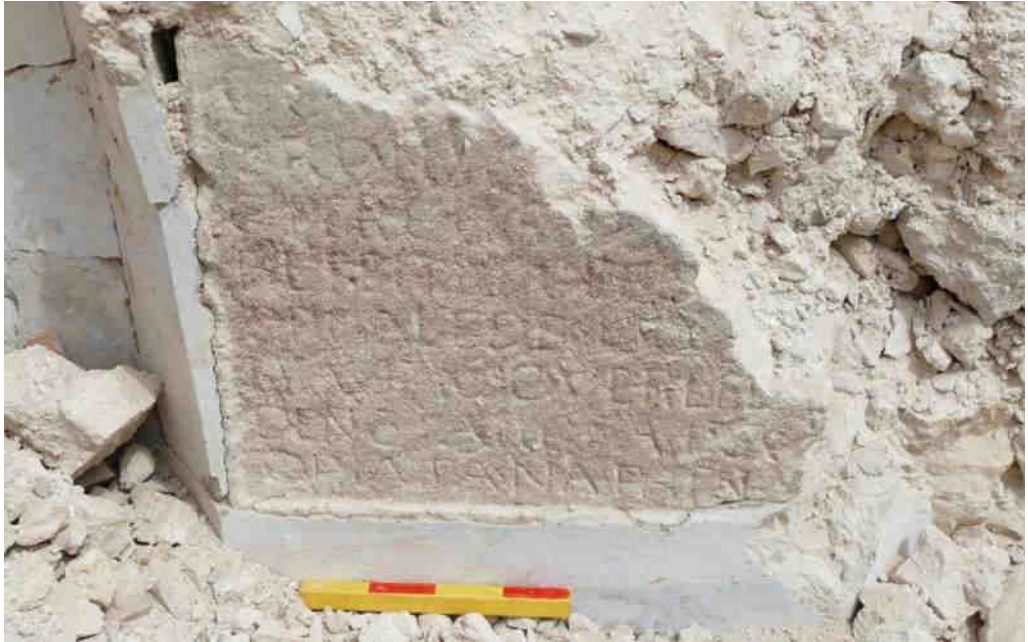
Figure 6: Damaged Dutch inscription identified, which was incorporated into the new Vestry, built into the space between the north and east wings of the original church construction.
