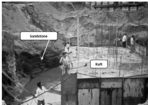
Figure 06: Exposed sandstone upon which raft is founded.
